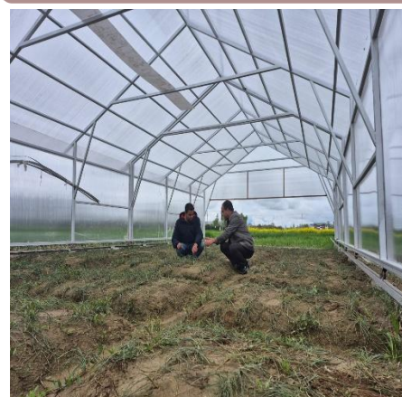
Fig.3: Installation of a rainout shelter for assessing the actual moisture requirement during corm development.
